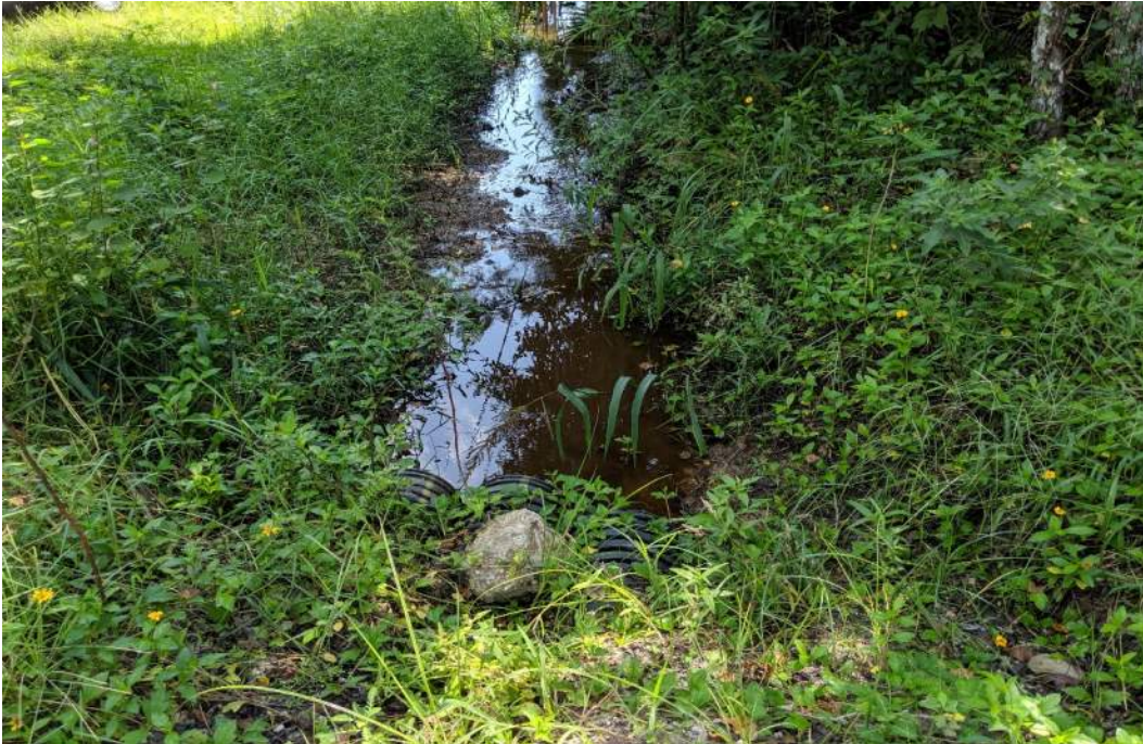
Photo 9: View of triple pipe sidedrain along the south side of Retreat Road taken in September 9, 2019.
