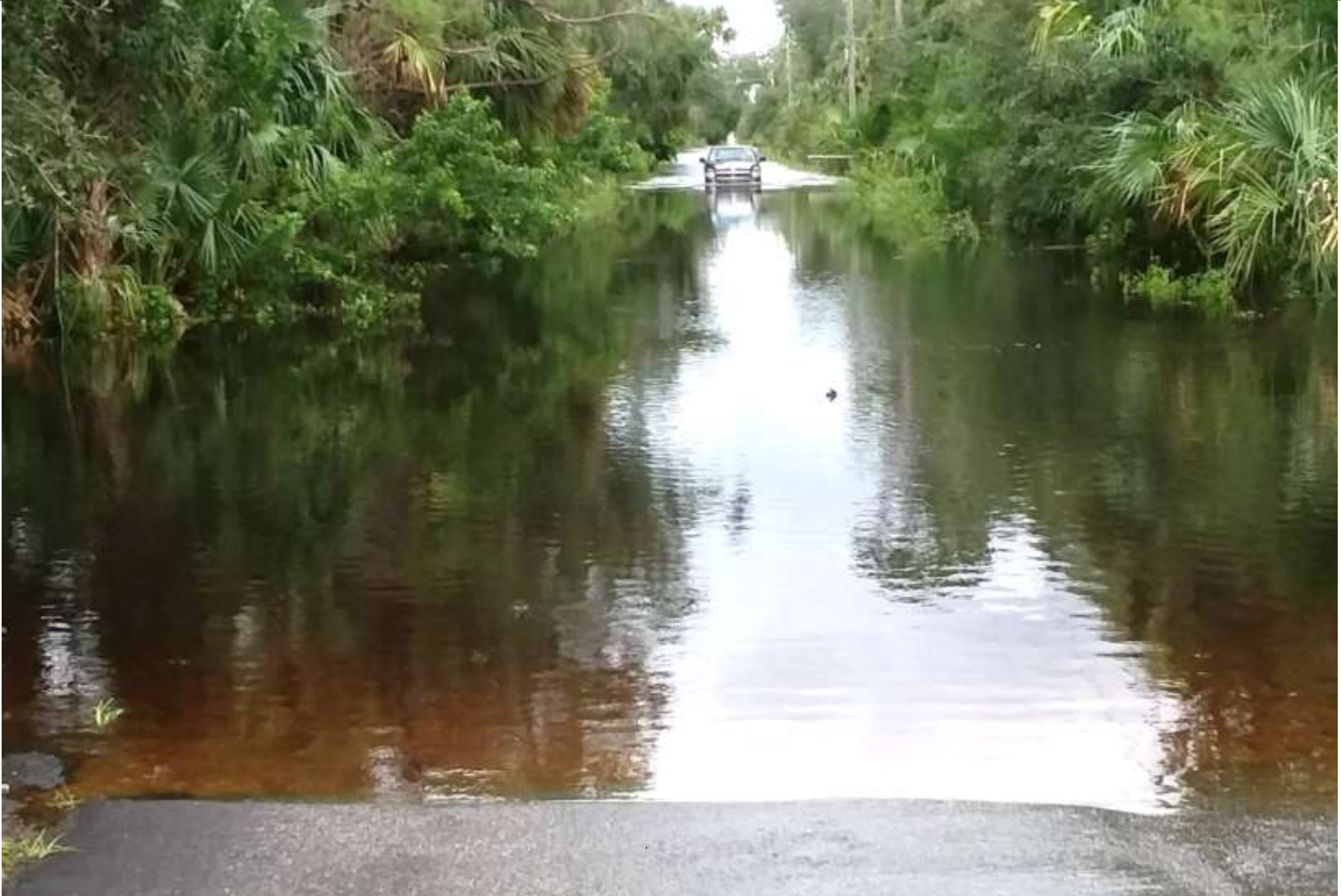
Retreat Road near Mullet Lake Park Road, Facing East – Hurricane Irma, 2017
