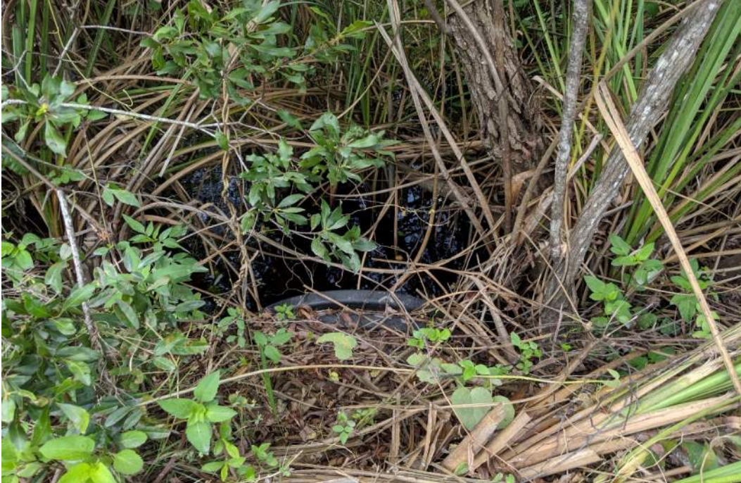
Photo 3: View a 24" CMP crossdrain along Retreat Road taken in September 9, 2019.
