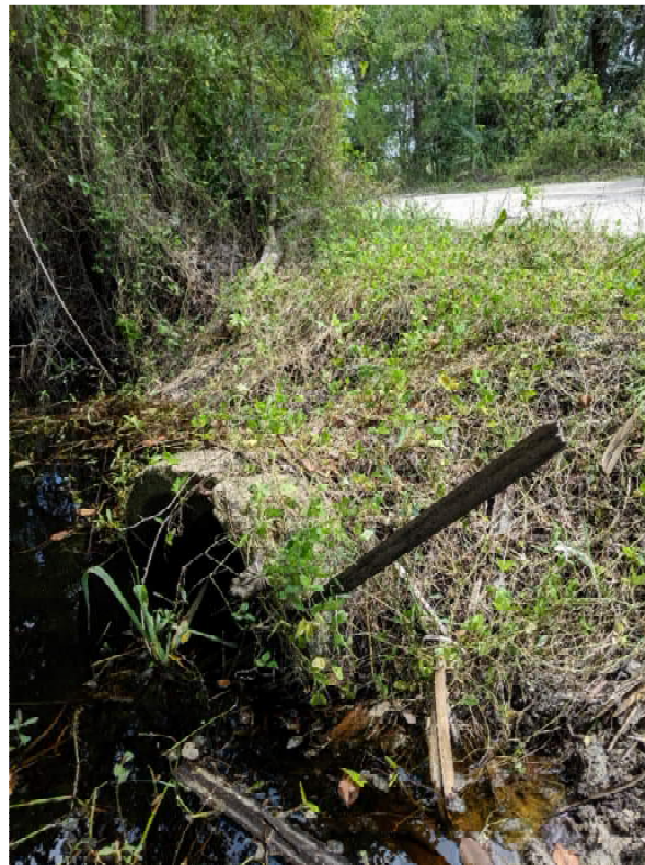
Photo 4: View a 24" RCP crossdrain along Retreat Road taken in September 9, 2019.
