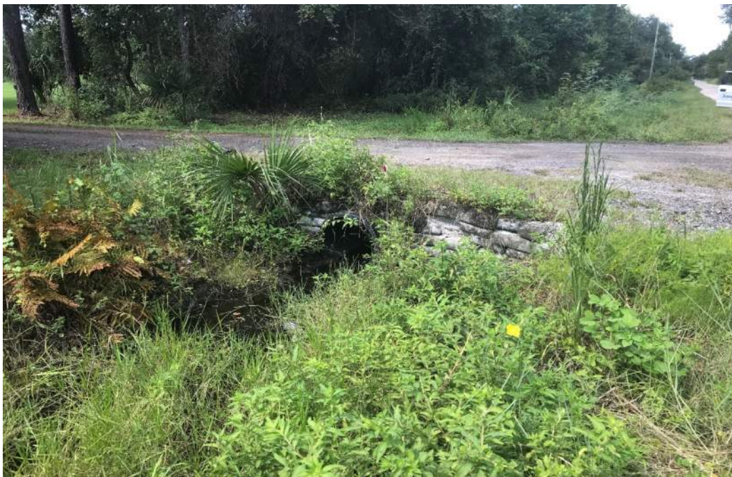
Photo 8: View of sidedrain along the south side of Retreat Road facing west towards MLPR taken in September 9, 2019.
