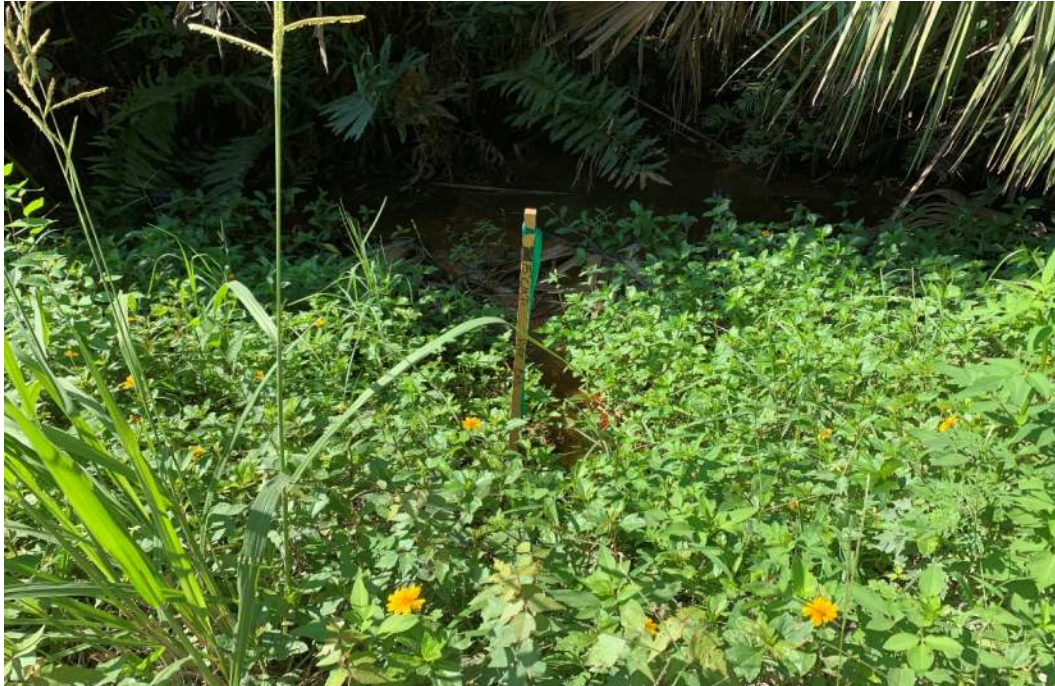
Photo 7: View of 15" CMP crossdrain along Retreat Road facing north. Pipe to be replaced in-kind taken in September 9, 2019.
